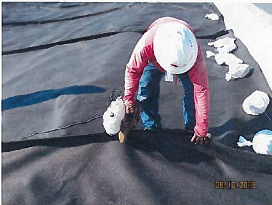
Sewing nonwoven geotextile seam (looking south).
