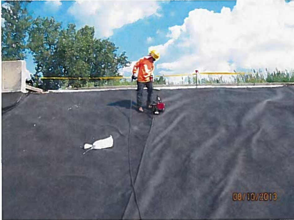
Fusion welding nonwoven geotextile seam (looking north).
