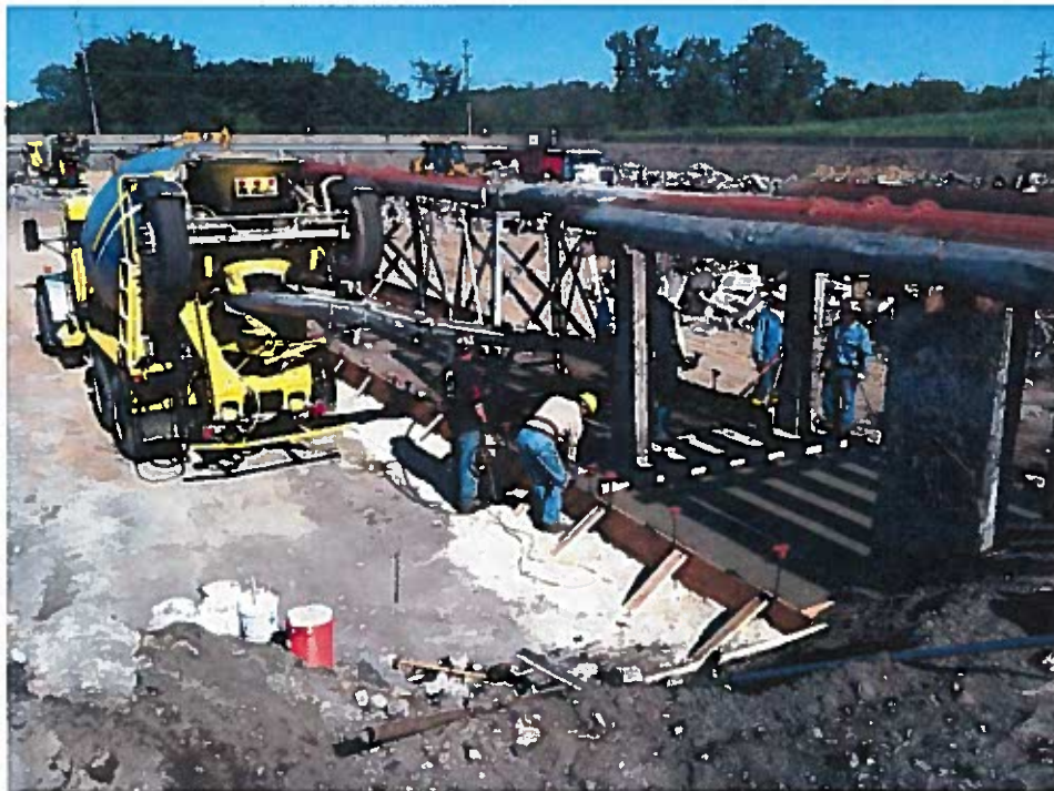
Placing and finishing concrete pad (looking northwest).
