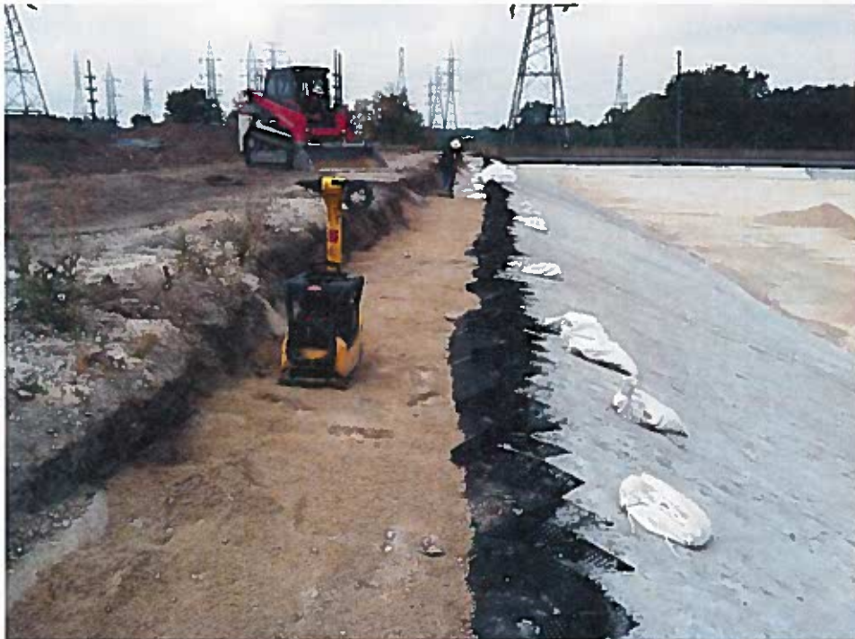
Brieser backfilling and compacting soil in the anchor trench (looking west).
