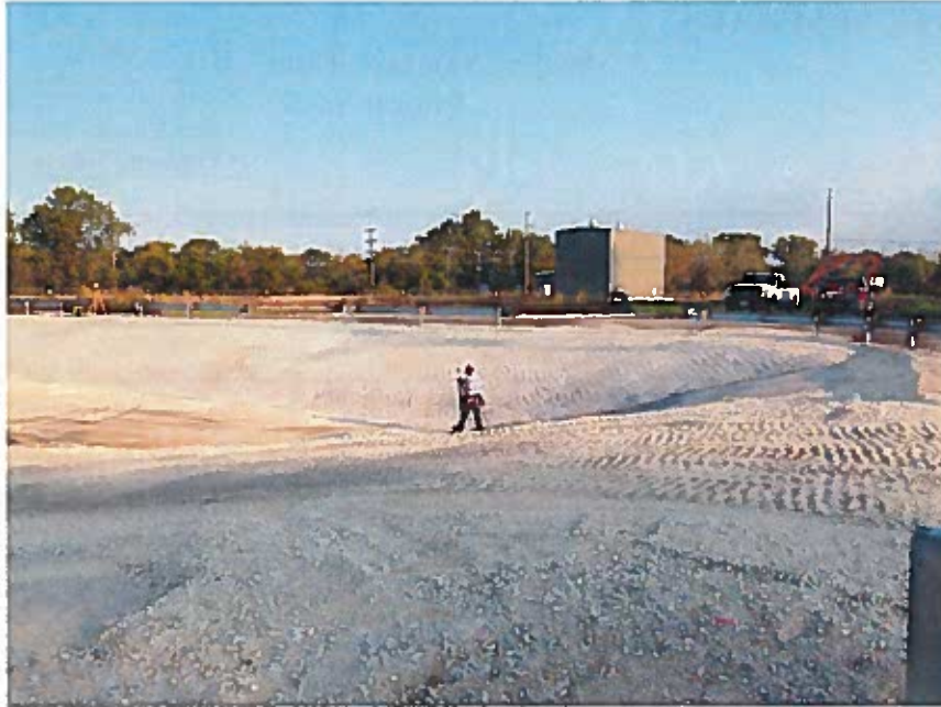
View of the ramp facing northeast
