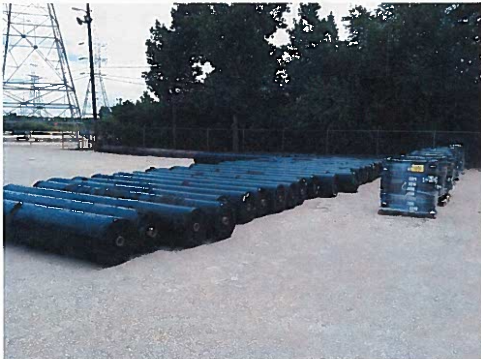
Geotextile and geocell staged in a gravel parking lot (looking north).
