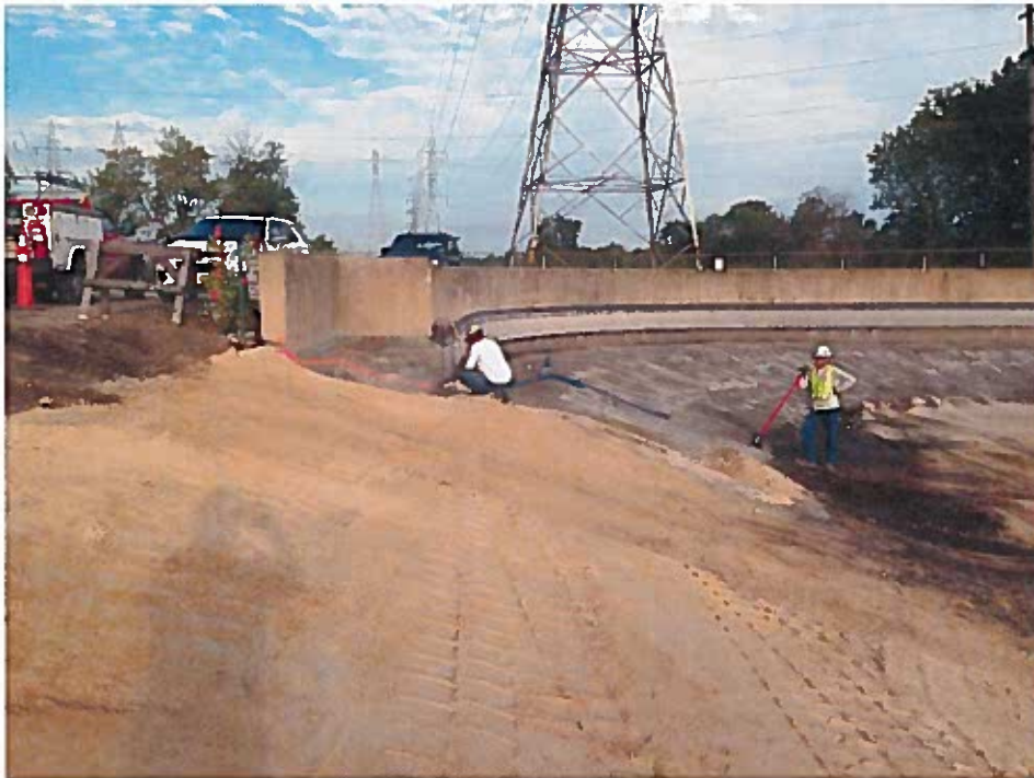
Brieser preparing subgrade for geosynthetics deployment (looking west).
