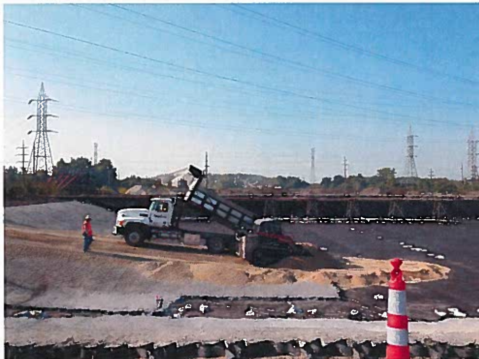
Placement of cushion layer over ramp and pond floor (looking south).
