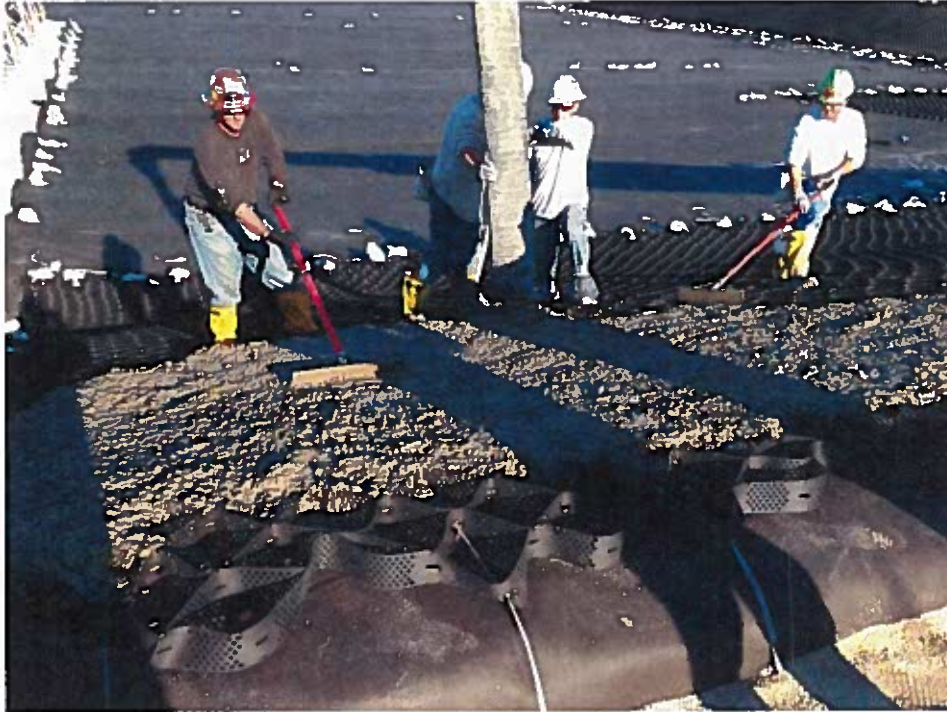
Concrete placement in geocell on the slope (looking west).
