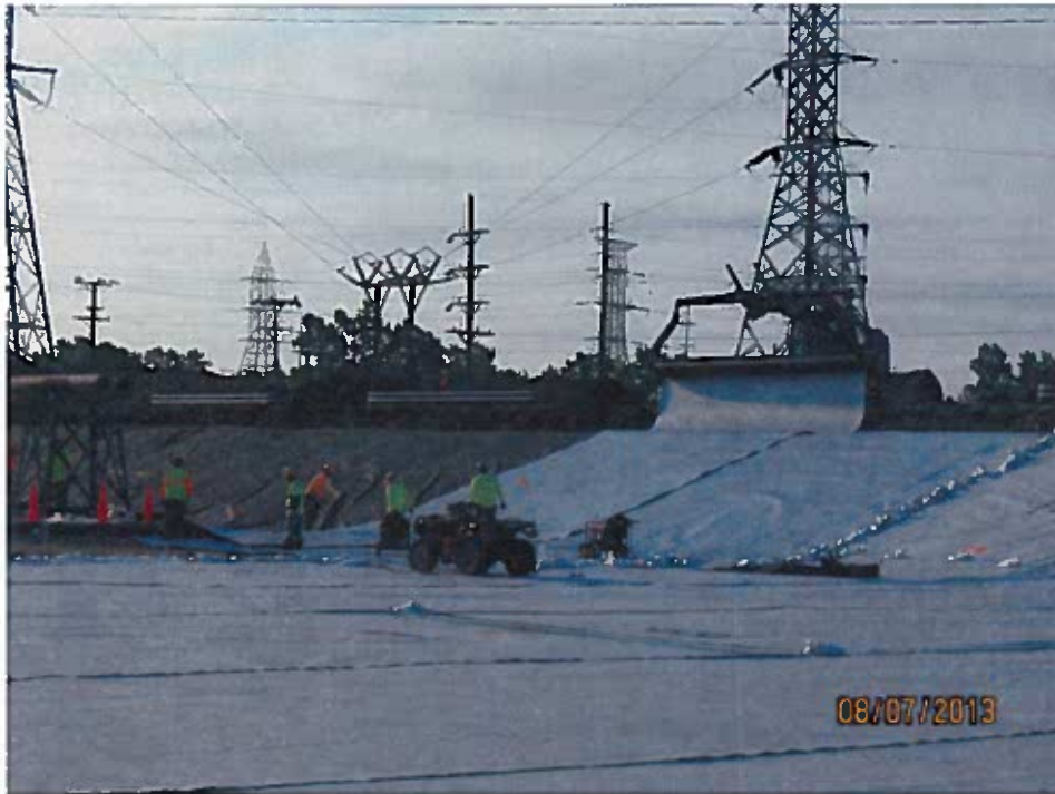
Geomembrane installation on the south slope (looking southeast).
