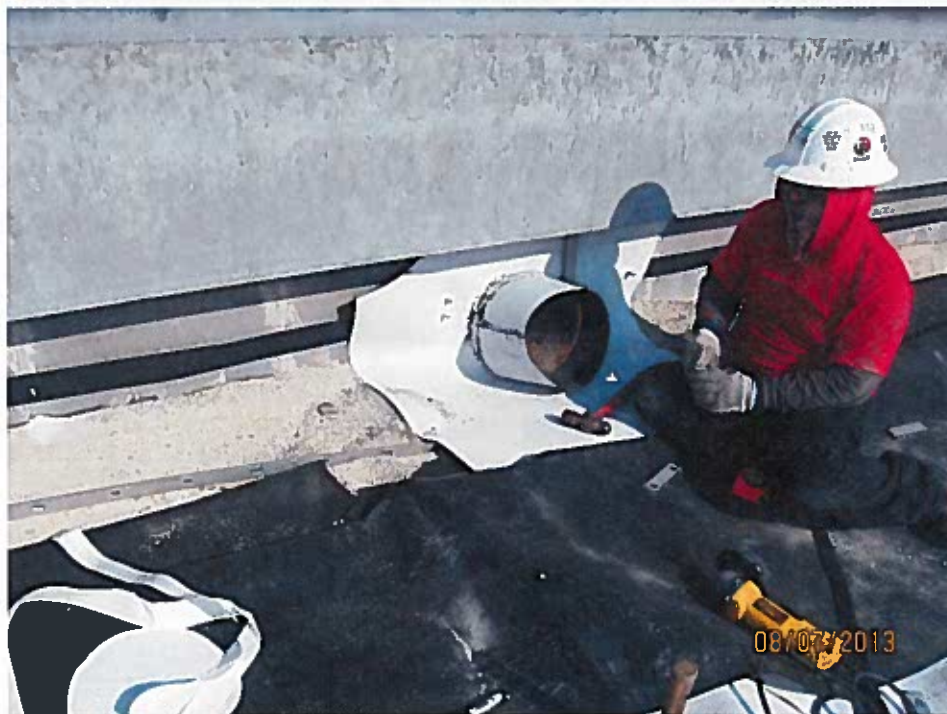
Pipe boot installation on pipe exiting the weir wall (looking northwest).
