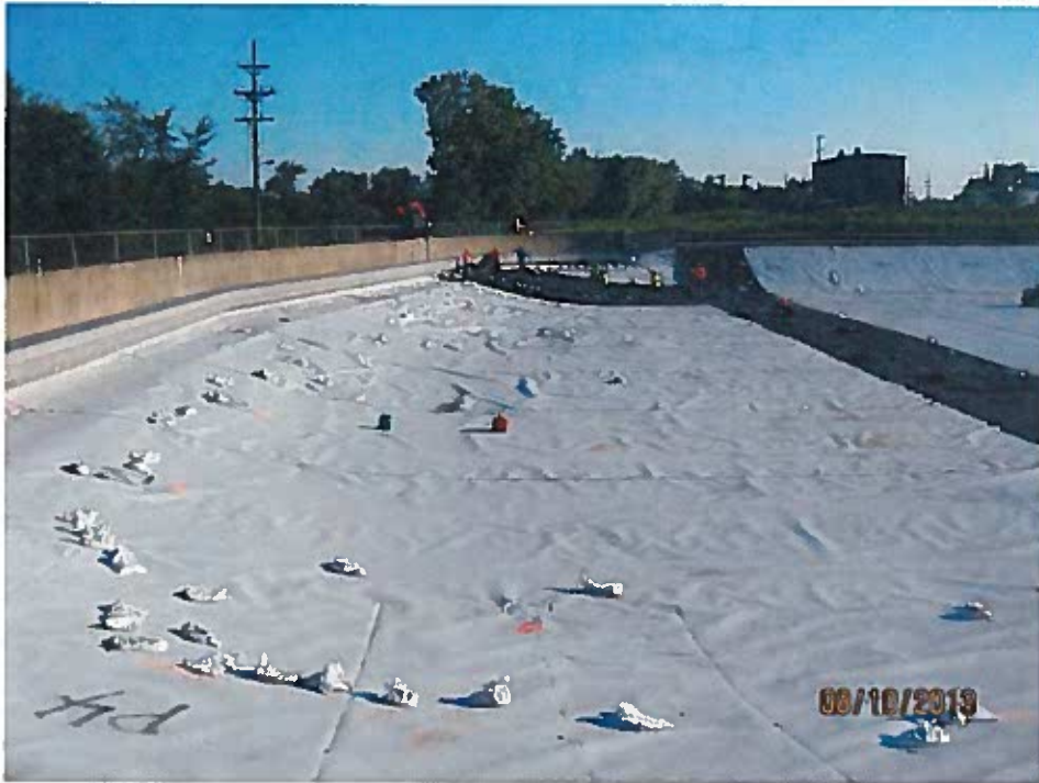
Installation of upper geotextile layer (installed over the geomembrane) (looking north).
