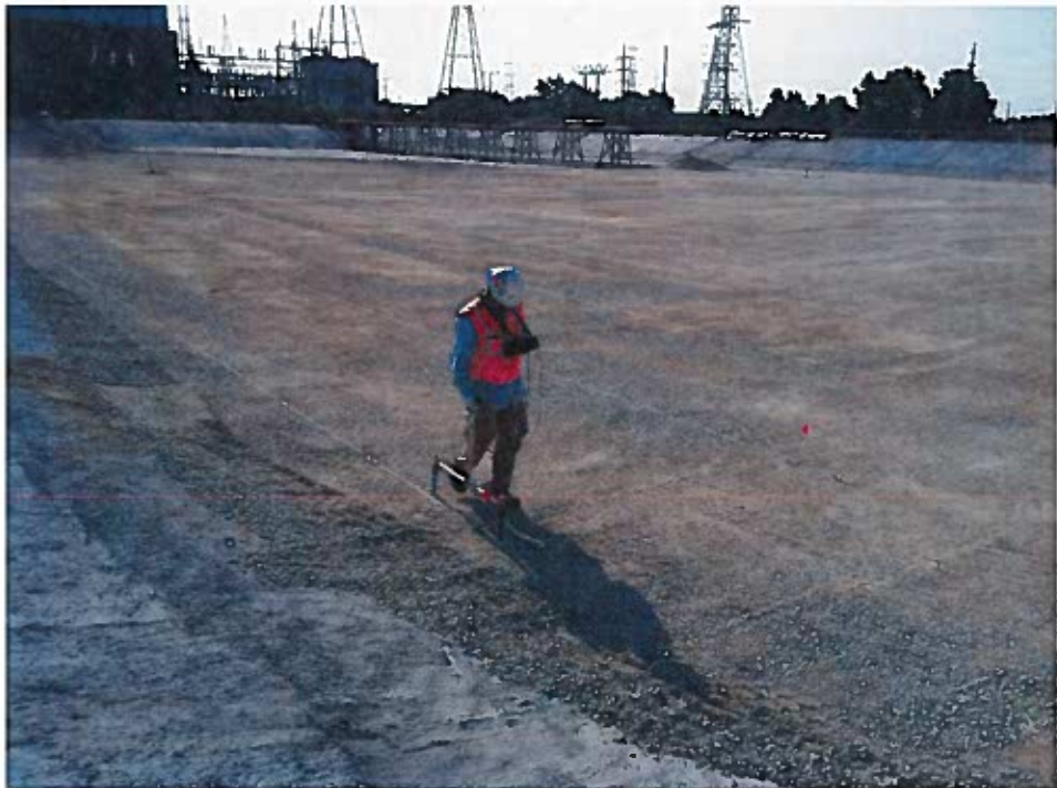
LLSI taking electric potential readings on the pond floor (looking southeast).
