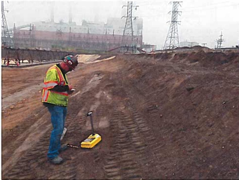
Density testing structural fill along the south slope (looking east).
