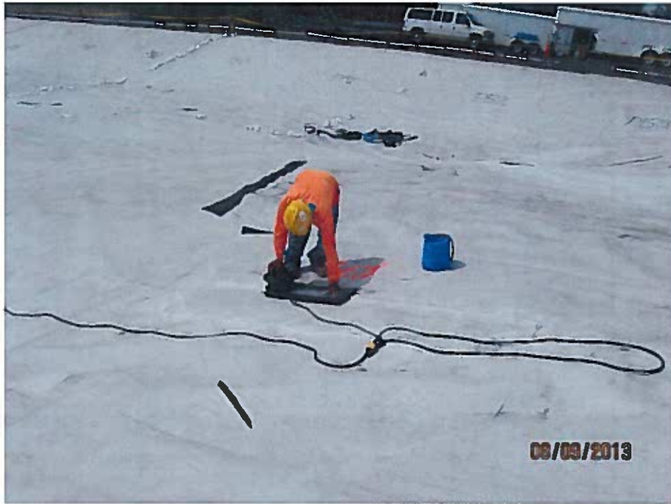
Vacuum testing geomembrane repair extrusion weld (looking north).
