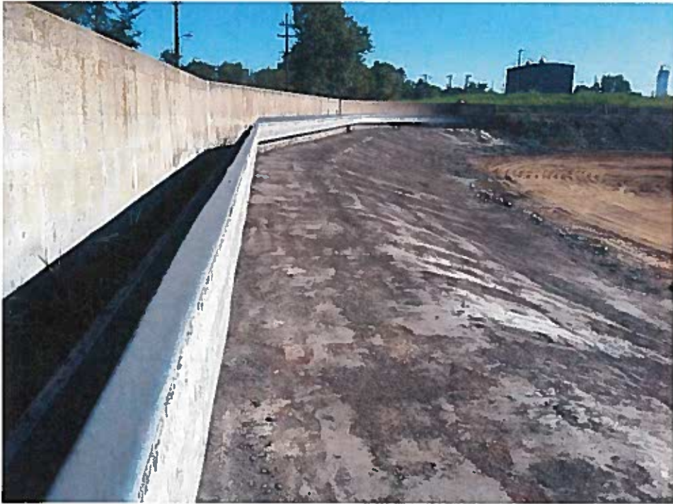
West slope graded in preparation for geosynthetics (looking north).
