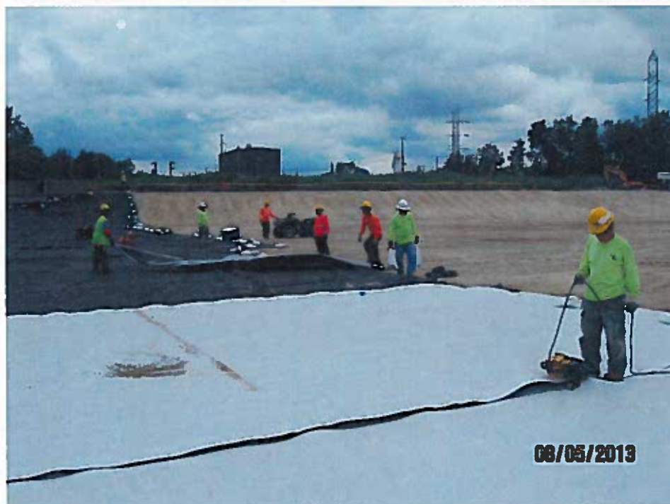
Fusion welding geomembrane seams (looking northeast).
