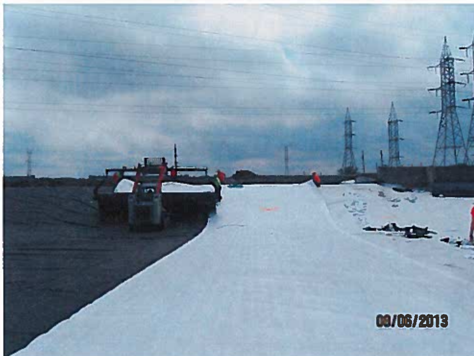
Geomembrane installation (looking south).
