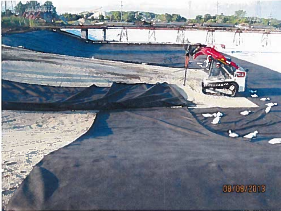
Geotextile installation (looking south).
