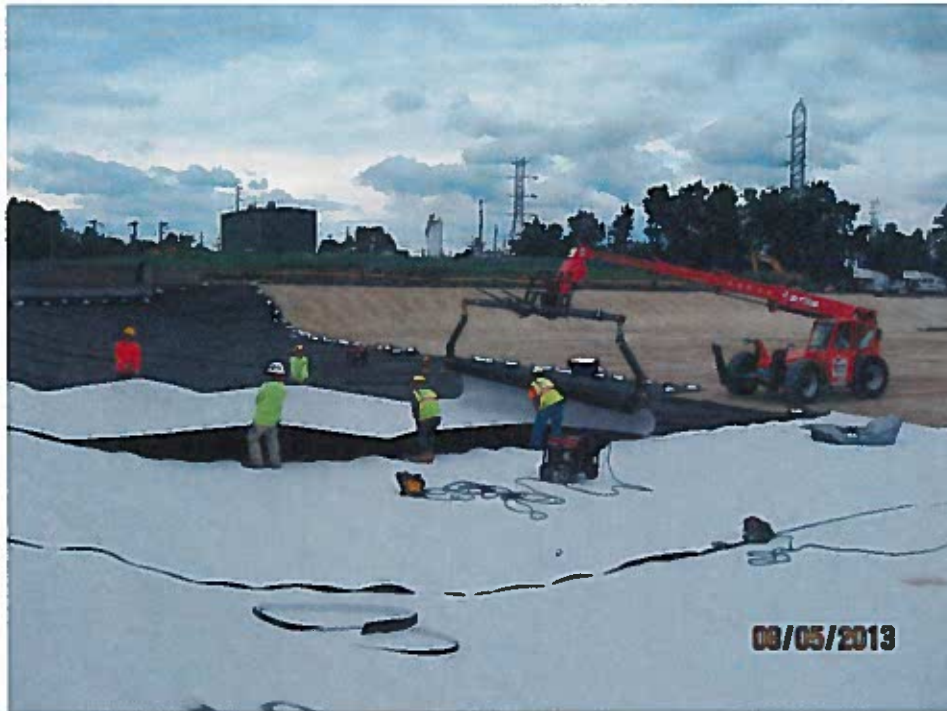
Geomembrane installation on the west end of the pond (looking northeast).
