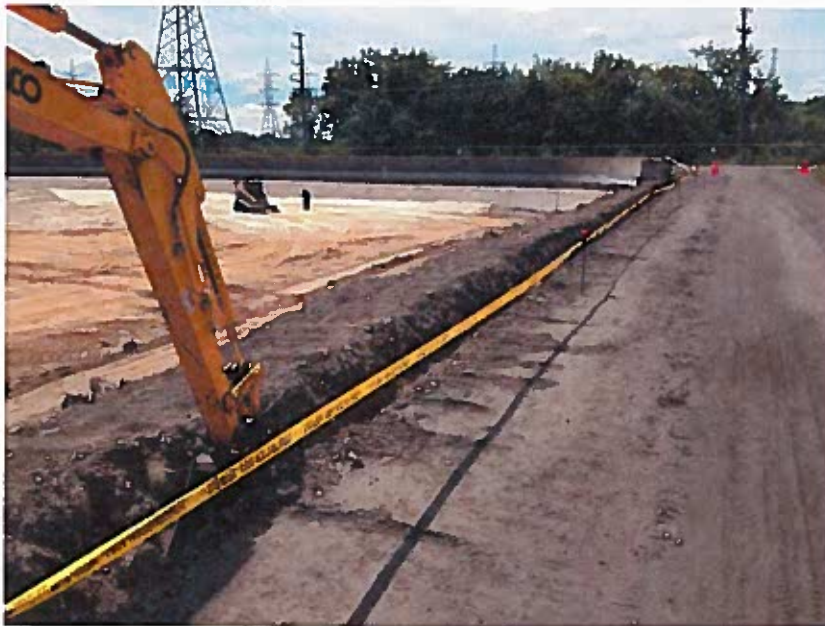
View of anchor trench excavation, facing west
