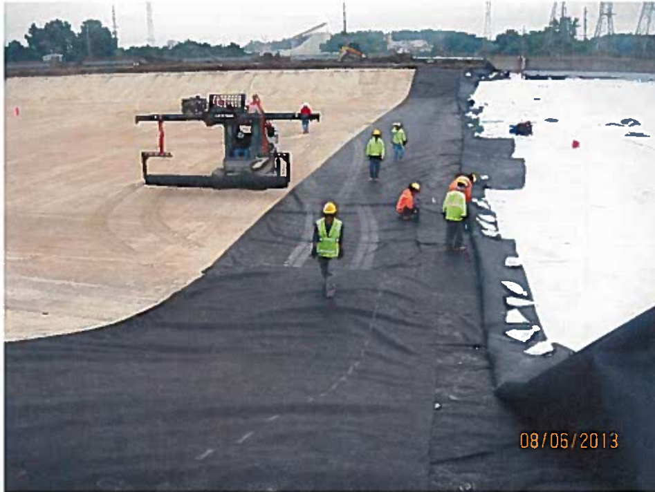
Geotextile installation (looking south).
