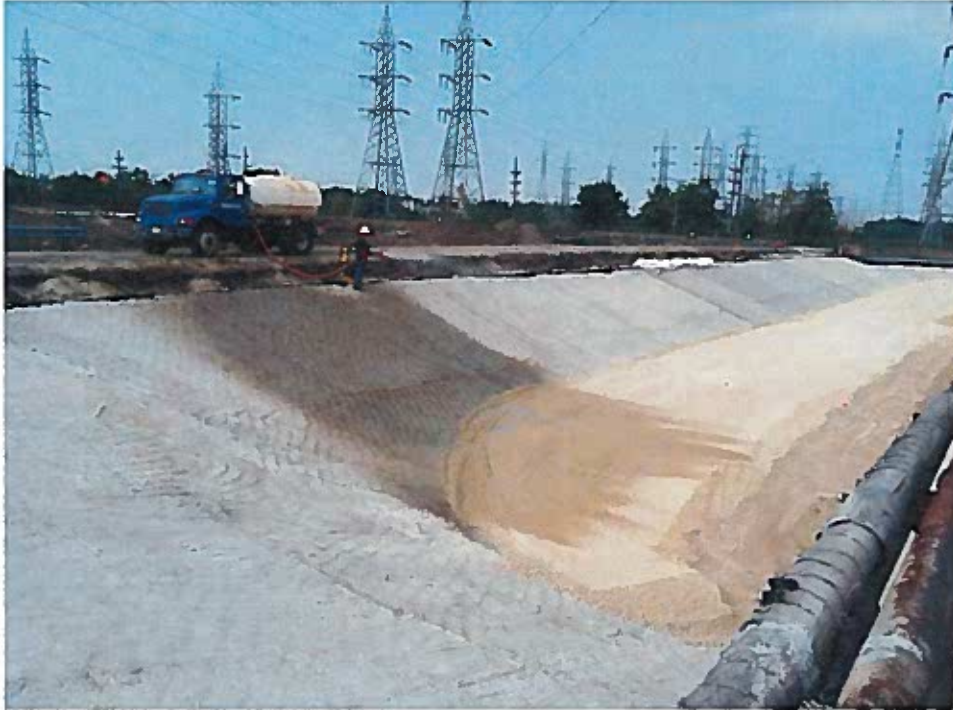
Brieser wetting the soil overlying the geomembrane for the liner integrity survey (looking southwest).
