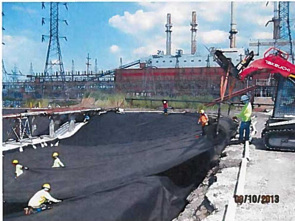
Geotextile deployment. PVC deadman staged along anchor trench (looking east).
