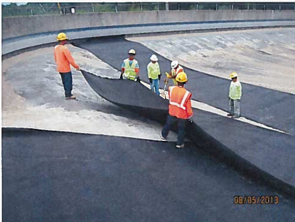
Geotextile installation on the west end of the pond (looking northwest).
