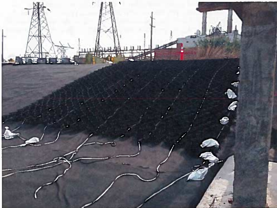
Geocell installed on the east slope (looking northeast).
